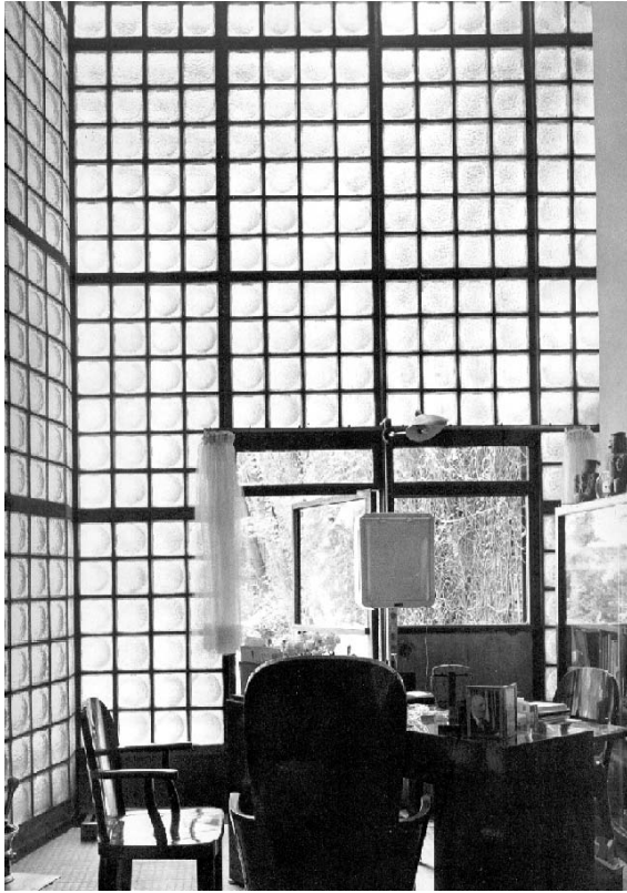
Figure 4. Translucent and transparent walls in an interior of P. Chareau's "Maison de verre". (Reproduced from GA No. 46, photograph by Y. Futagawa).
